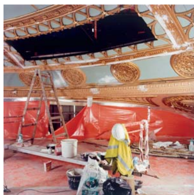
Work in progress at the Royal Opera House
