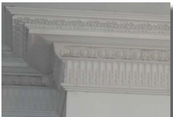
After: Restored cornice in Mr. Boldt's Suite
