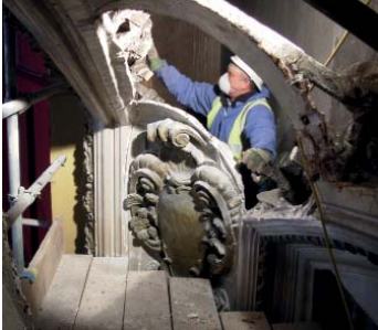
David Harrison dismantling the Arch
