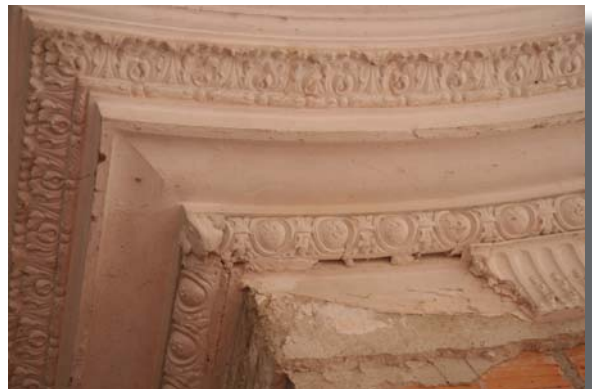
Before: Cornice in Mr. Boldt's Suite
