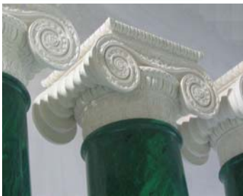
These Stunning Malachite Scagliola Columns and plaster Capitals were introduced to the Entrance Hall design instead of the original Verde Antico columns of the ante-room at Syon House, Middlesex UK
