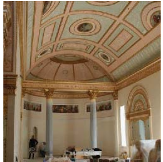
The installed replica interior of the Ornamental Plasterwork and Paintings of the Great Library at Kenwood House in Hampstead, London
