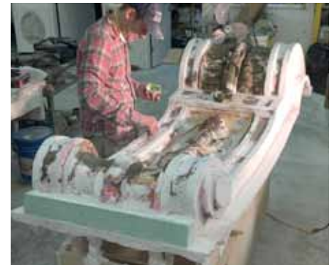
Pictured below is Jim Meade restoring a large corbel.
