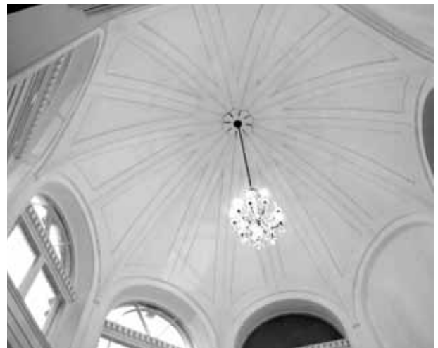
Architect's drawing for an octagonal vaulted ceiling (left) and (above) the finished ceiling as manufactured and installed by Hayles & Howe.
